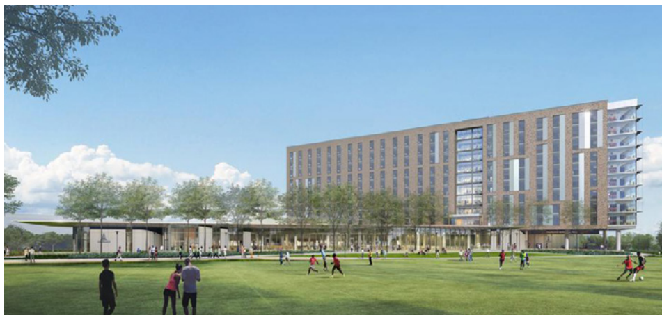
Rendering shows the Thurgood Marshall Project, a new student housing and dining project, planned at Morgan State University.
