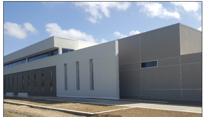
Top photo: UVI Medical School Classroom Building, St. Thomas Campus Bottom photo: UVI Medical School Simulation Center, St. Croix Campus
